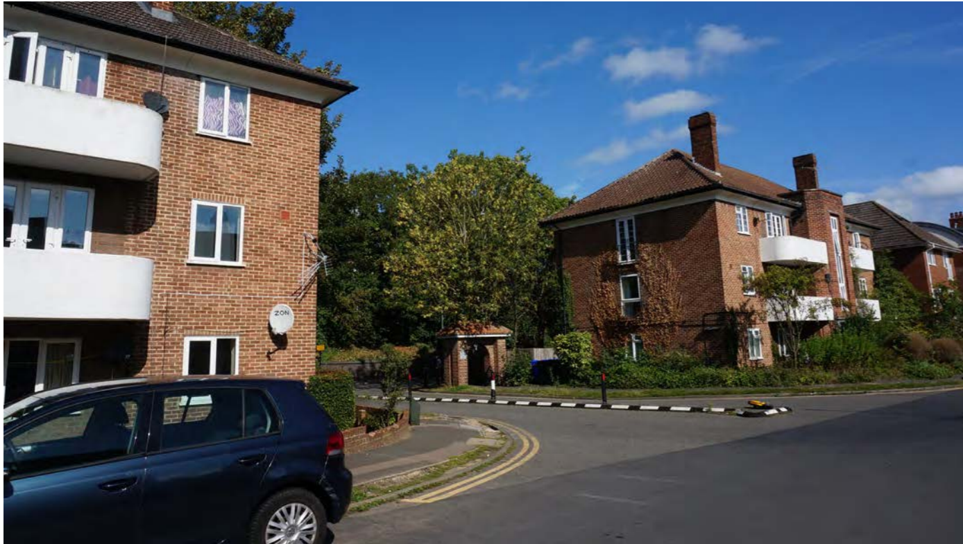
View S7 - Existing View
