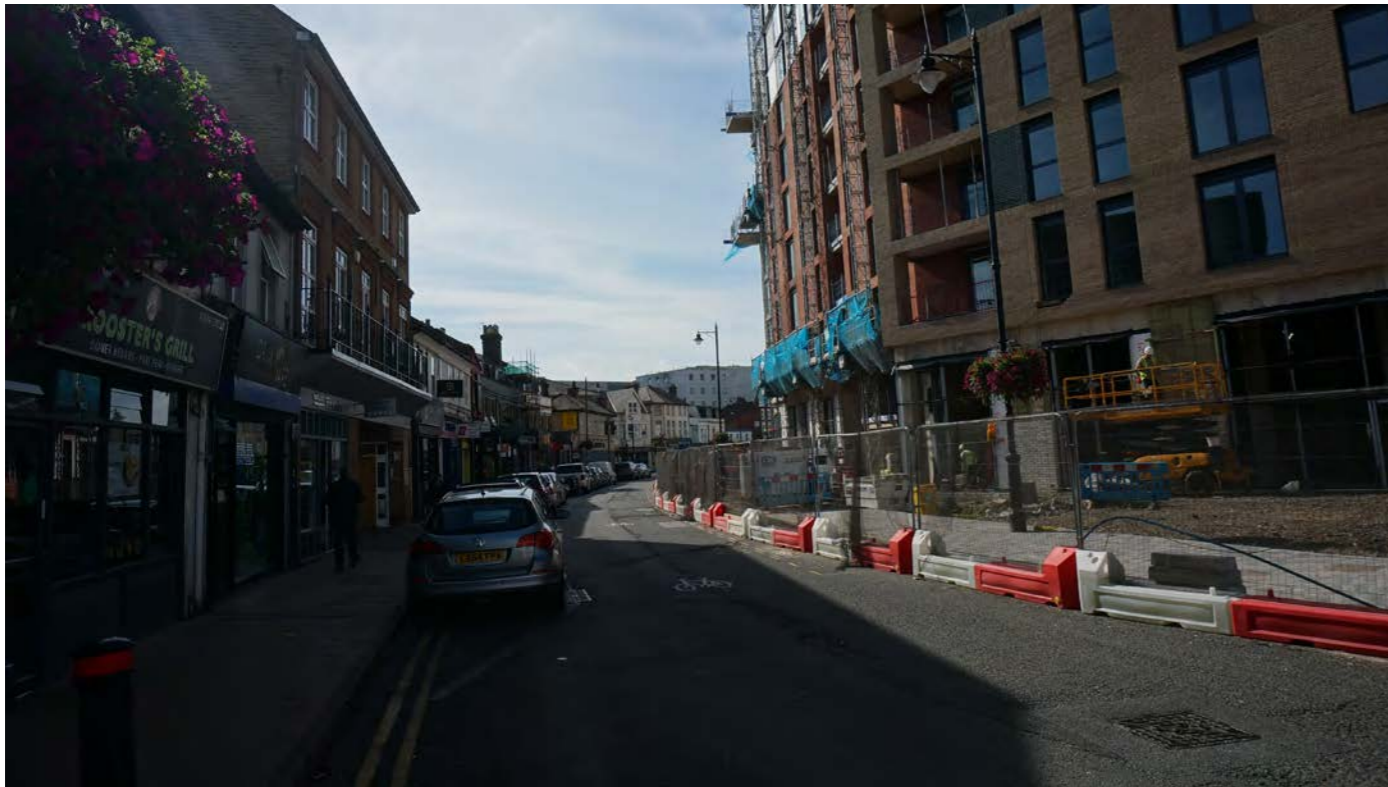
View S2 - Existing View
