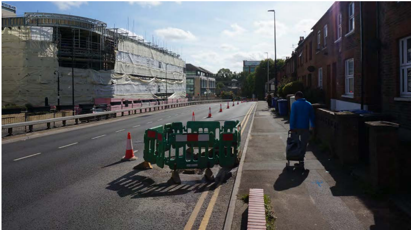
View S4 - Existing View
